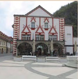
Kamnik, façade of the house at Maistrova 2 (1954)
