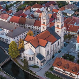
Ribnica, bell tower of the Church of St. Stephen (1956)
